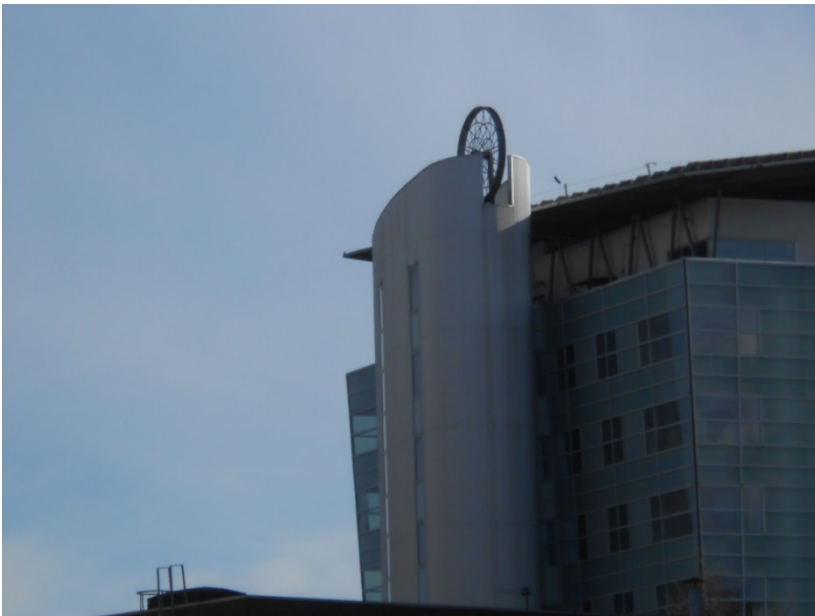
Fig. 1. The elevator wheel atop the town hall in Kerkade.
